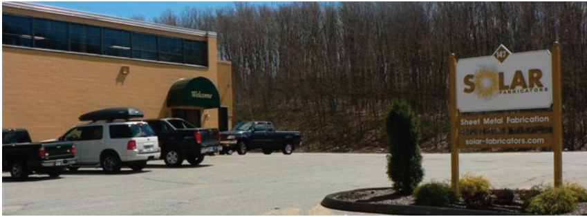
FIGURE 3 In setting up Solar Fabricators down the road from Seconn, Marelli and his team cleaned up the old Crown Manufacturing building and invested in new equipment, lighting, landscaping, and paint. By the beginning of this year, the new fab shop was ready to take on small projects, such as repairing snowplow blades, that don't fit Seconn's business model.
